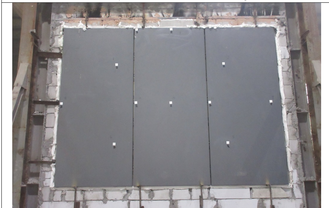
The unexposed side after the test
